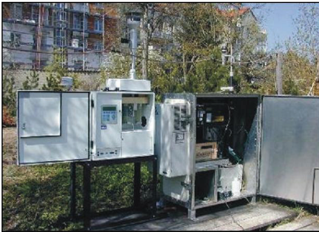
Figure 3.10 Aerosol monitoring station in Augsburg, Germany
