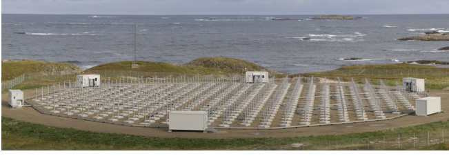
Figure 3.1 MAARSY is an active phased array with 433 antennas, located at Andenes, Norway, above the polar circle. Photo: Ralph Latteck.
