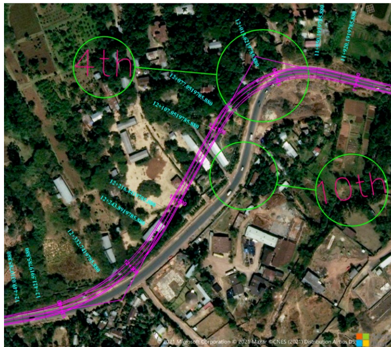
Figure 21: The fourth-ranked hazardous road segment
