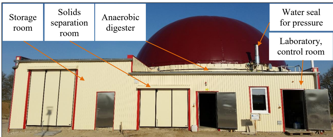
Figure 9.5: Photo of the anaerobic digester and operation buildings at site Fahrbinde
