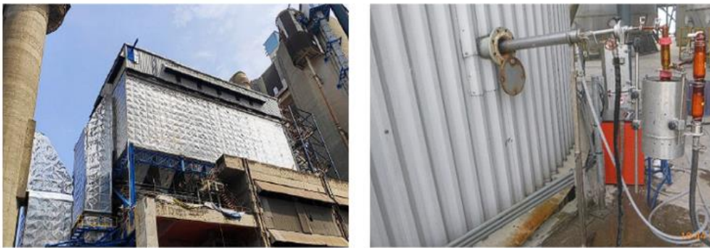
Figure 8. 2 Bag filter (right) and CEMS (left) (Indocement, 2023b)
