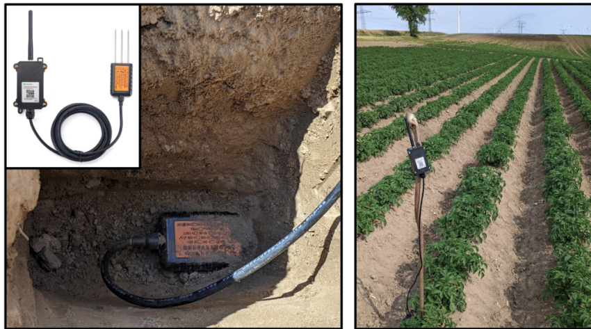
FIGURE 4.1: Dragino LSE01 soil moisture sensors installed in the field in Kassow, Germany.
