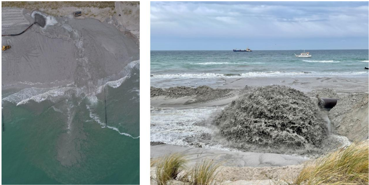
Fig. 2 Photos of the sand nourishment in Ahrenshoop. Sand is nourished onto the beach with water through a pipe system from a ship and then distributed from there using heavy machinery. Left picture taken by Jan Tiede, right picture taken by StALU MM.
