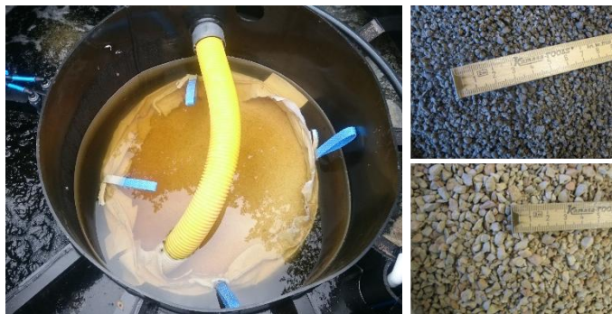
Figure 2: Left: A phosphorus filter integrated into an on-site package plant for domestic wastewater treatment. Right: Examples of filter materials used in phosphorus filters. Upper right: Filtralite® P; lower right: Polonite®.
