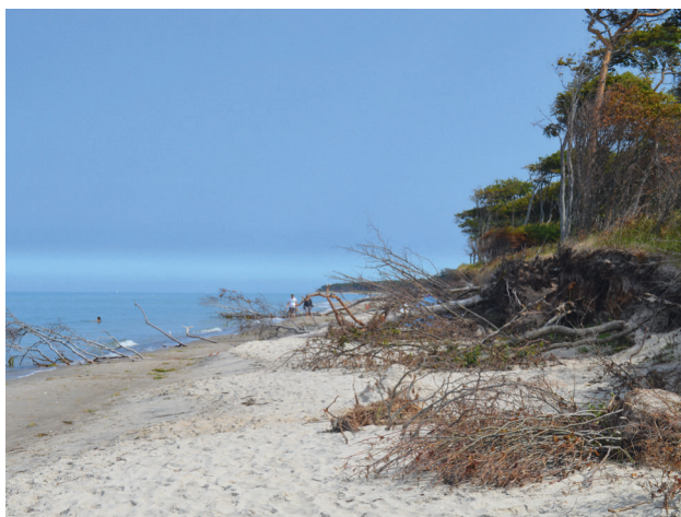
Figure 27 Storm damage on beach (© EUCC-D)
