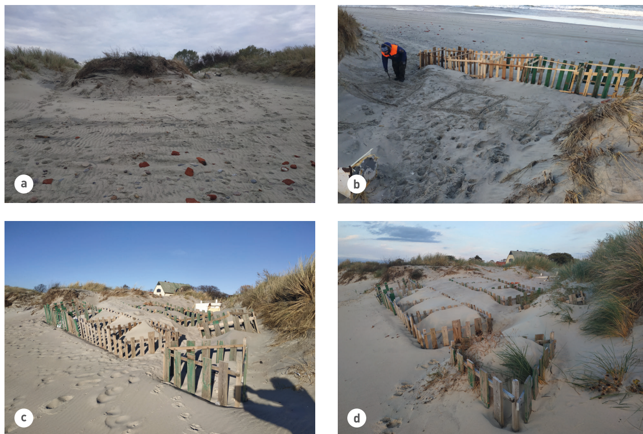
Figure 4.20. Experiment with wooden cells on the shore of the Vistula Spit: (a) the selected site (the right passage through the foredune), (b) construction process, December 2019, (c) after the wintertime, March 2020, (d) after the summer, with some grass already grown in triangular cells, which were preliminarily filled with beach wrack, October 2020. Photos: B. Chubarenko.
