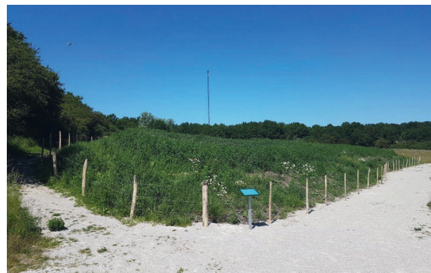
Photo VIII Pilot Installation of a Biocover in Köge municipality, photo: J. Engelbreth Larsen.
