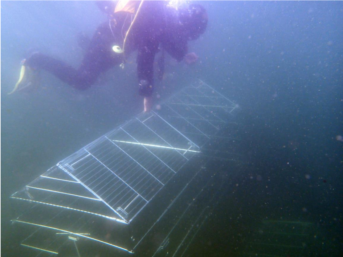
Fig. 5: Installation of enclosure.
