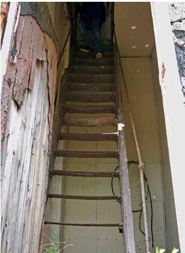
Abb. 33. Insel Ruden, Lotsenwachturm, Innentreppe, EG, 2021, (LAKD M-VILD, J. Kirchner).
